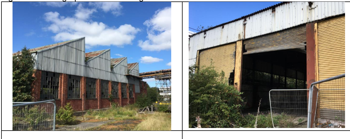
Figure 2. Photographs of the building
